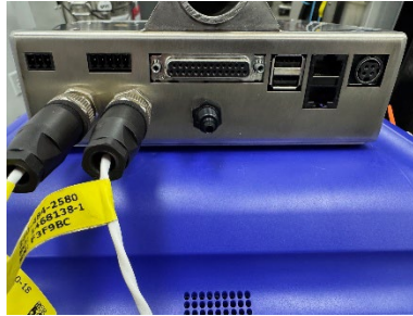
Figure 4. Temperature Sensor Connection to CryoVerse Connect
