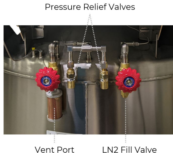
Figure 21: Vent port, dual Pressure relief valves, LN 2 fill valve
